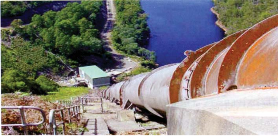
A cleaning trial of the penstock supplying the 32-mw Wilmot project improved production by 1 gigawatt-hour. This improvement met Hydro Tasmania's expectations, so other penstocks were scheduled for similar cleaning.
