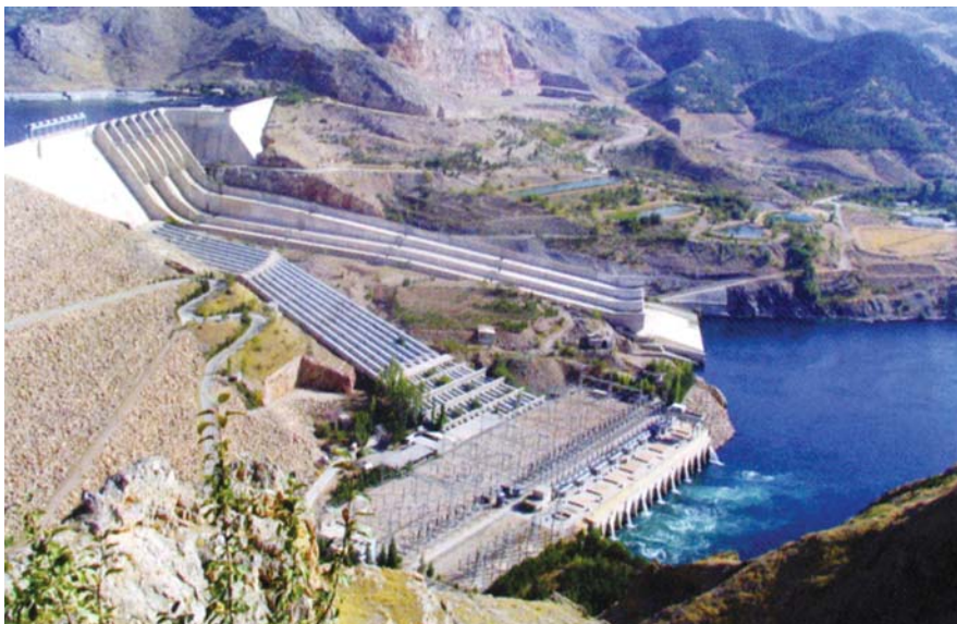
The 1,350-mw Keban project on the Euphrates River in Turkey was chosen as the best rehab and uprating project in the country, as a result of using the framework developed by Electricite de France.
